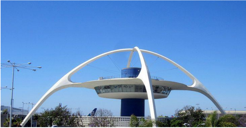
fig. A. Theme Building, exterior. Two parabolic arches circumventing at the top and the Encounter Restaurant & Lounge in the middle. Photo source: myarchetypes.wordpress.com
