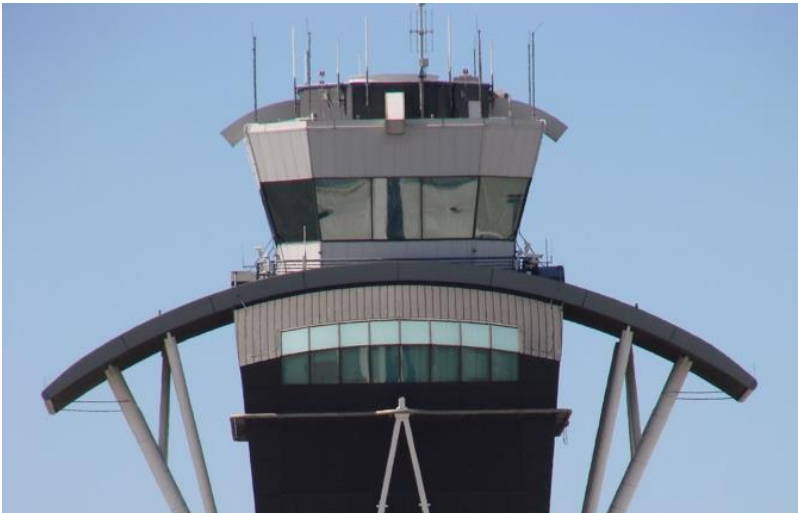
fig. D. LAX control tower, exterior. Photo taken by John Murphy.
